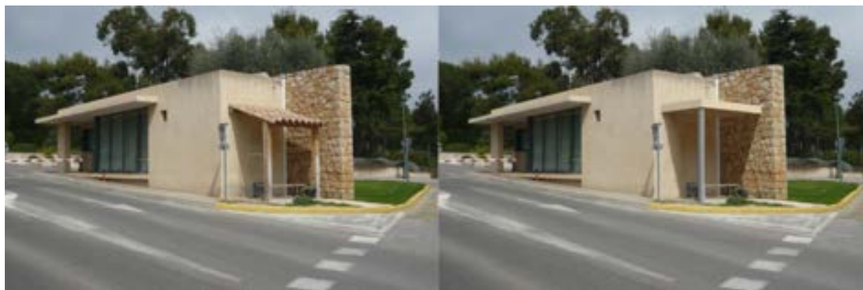
Abri bus existant
